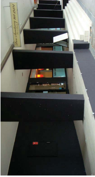
02 Struggling retail shops elevated from footpath level
