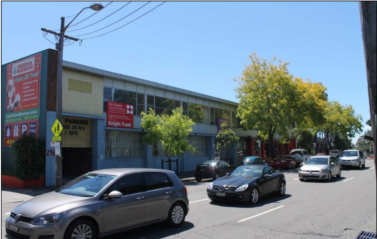
Figure 6: The site (northern lot) as viewed looking west from Botany Road.
