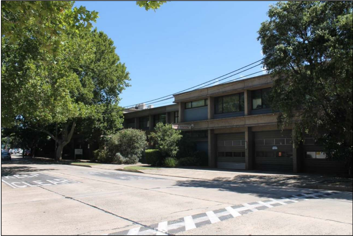
Figure 12: Part of the NSW Fire Brigade Training College, fronting Wyndham Street to the west
